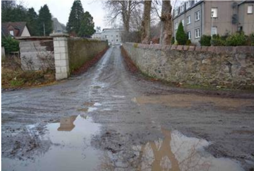
Photo 2 South Avenue – East boundary of application toward the A93 junction
